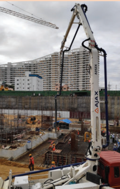
AJAX boom pump in action. Site: Commercial Building – Embassy Group – Manyatta Tech Park, Bengaluru.
