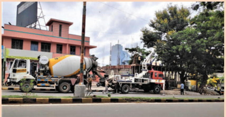
AJAX boom pump in action at UltraTech RMC. Site: Residential Building, Mysore
