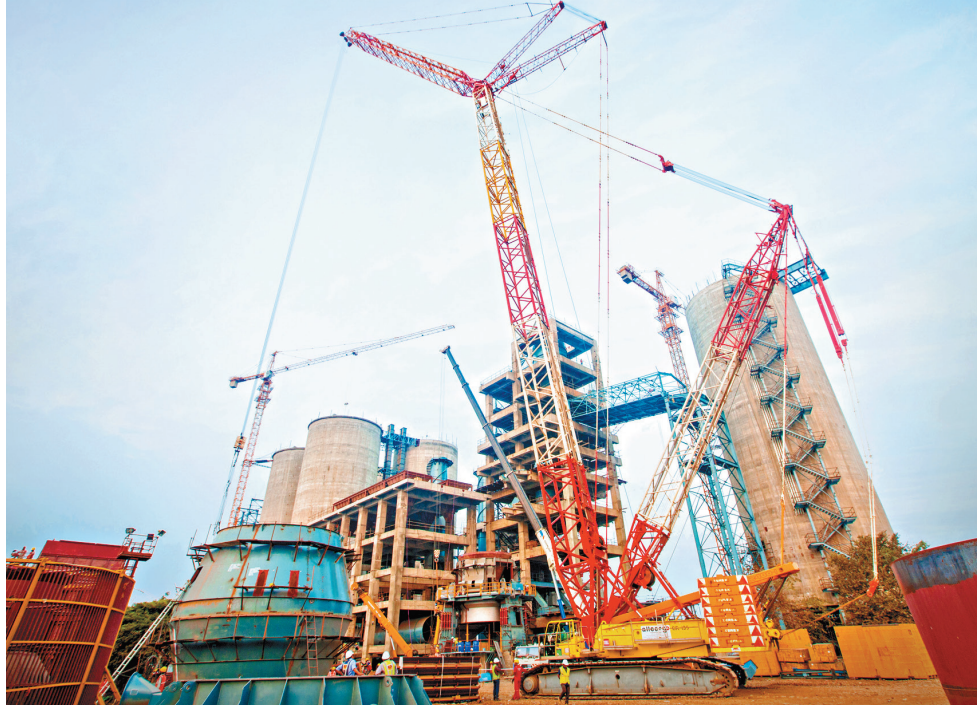
400 MT Demag CC 2400-1 at UltraTech Cement, Madhya Pradesh for preheater and kiln shell erection.
