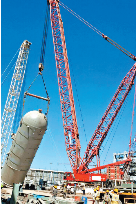
750 MT Liebherr LR 1750 at RIL Jamnagar for heavy vessels lifting.
